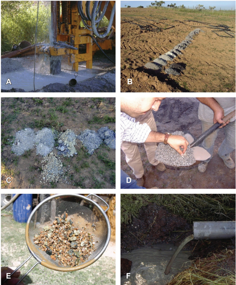
Plate 14 Drilling in hard rocks (A). Steps during the construction of the well: drill cuttings taken every 3 m (B), a section showing material which indicates a probable fracture (C), close analysis of the cuttings directly picked from the well during drilling (D), or after washing the cuttings with water to clean away dust (E), and observing the flow coming from the well during drilling, using compressed air directed to the bottom of the well (F). (see Fig. 4.12).
