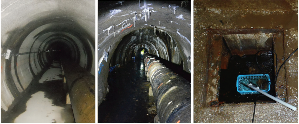
Plate 37 Left: a part of the tunnel excavated by boring machine with wet and dry strips visible; Middle: a part by drill-and-blast method, shotcrete covered, with more visible inflow; Right: an uncovered shaft to the collection canal (conductivity measurement during the dilution experiment). (see Fig. 15.2).
