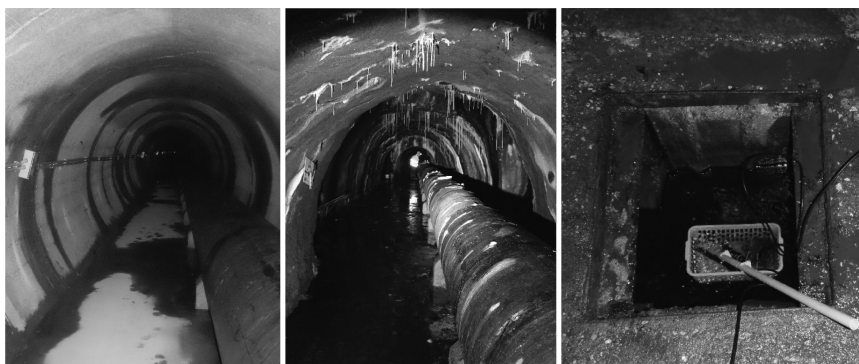
Figure 15.2 (Left) a part of the tunnel excavated by boring machine with wet and dry strips visible, (Middle) a part by drill-and-blast method, shotcrete covered, with more visible inflow, (Right) an uncovered shaft to the collection canal (conductivity measurement during the dilution experiment). (See colour plate section, Plate 37).
